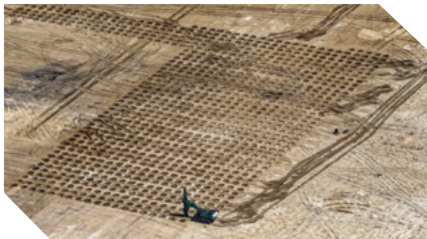
Jurong Island land preparation, Singapore
