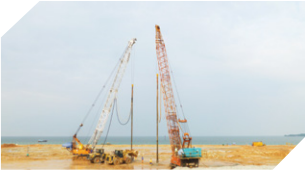
Karimun Petroleum Storage Terminal
