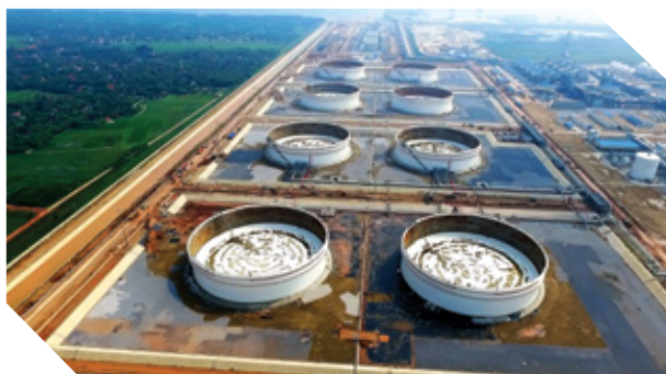
Nghi Son Refinery, Vietnam
