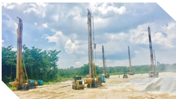
Ground Improvement for Expressway, Malaysia
