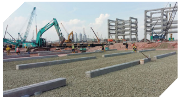
Petrochemical Complex, Malaysia
