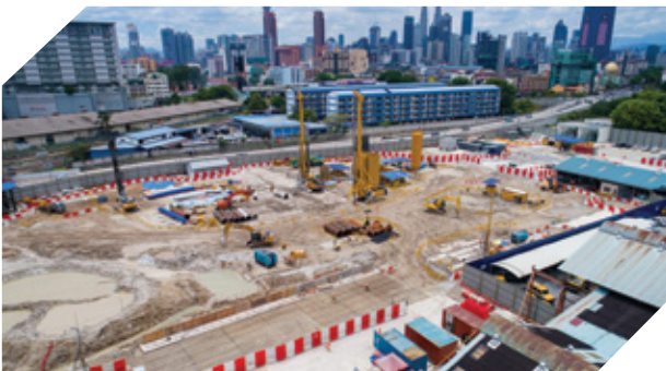
MRT Retaining System, Malaysia
